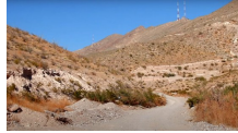
Paliades Stormwater Drainage project will increase dam capacity and control stormwater runoff.
